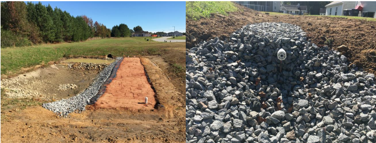
Figure 2. Littoral shelf filter following construction (left) and underdrain (right).
