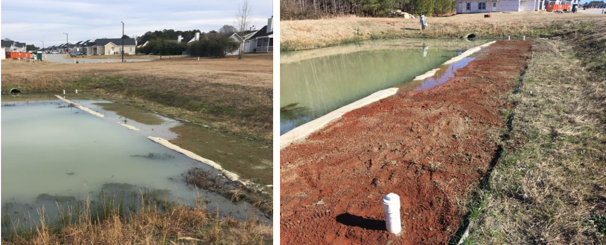
Figure 4. Biological blinding of the shelf filter observed at the Sapphire pond (left) remedied by raking of the filter surface (right).
